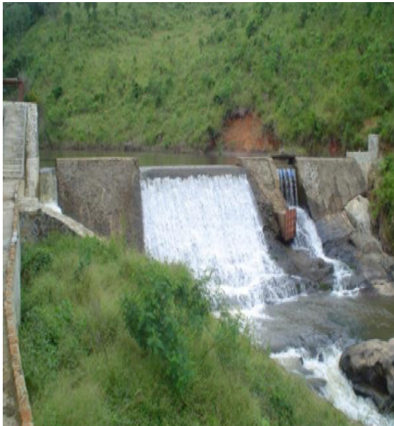
Mwenga Hydro Power Station in Mwenga Village supplying electricity to About 42 Villages
